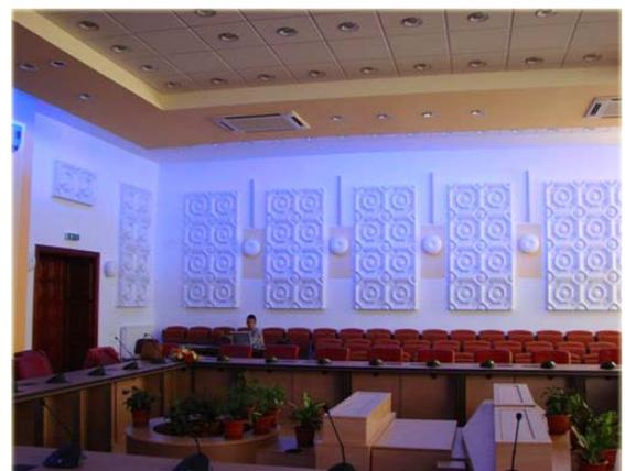
■ The solution for the specific recording rooms, Music Halls or TV plateau situations, rooms for live music of any dimensions is: many patches of at least 8 (in a 2x4 matrix) or 9 (in a 3x3 matrix) grouped R1 must be periodically / symmetrically mounted , if possible on all lateral walls and sometimes on ceiling.
